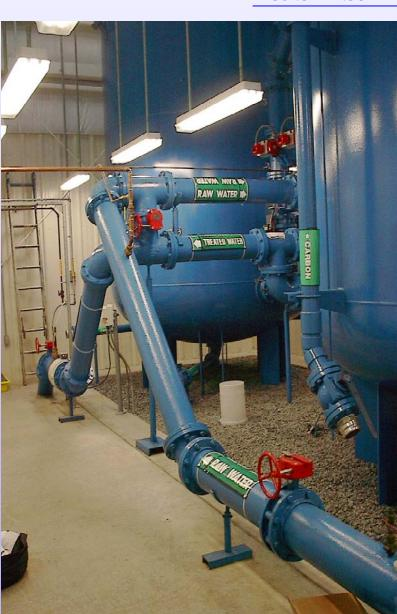
Our work for Plymouth Water Division included design and services during construction for a new water treatment facility. Treatment removes ethylene dibromide (EDB) from groundwater from an existing 1.5 mgd supply well.
